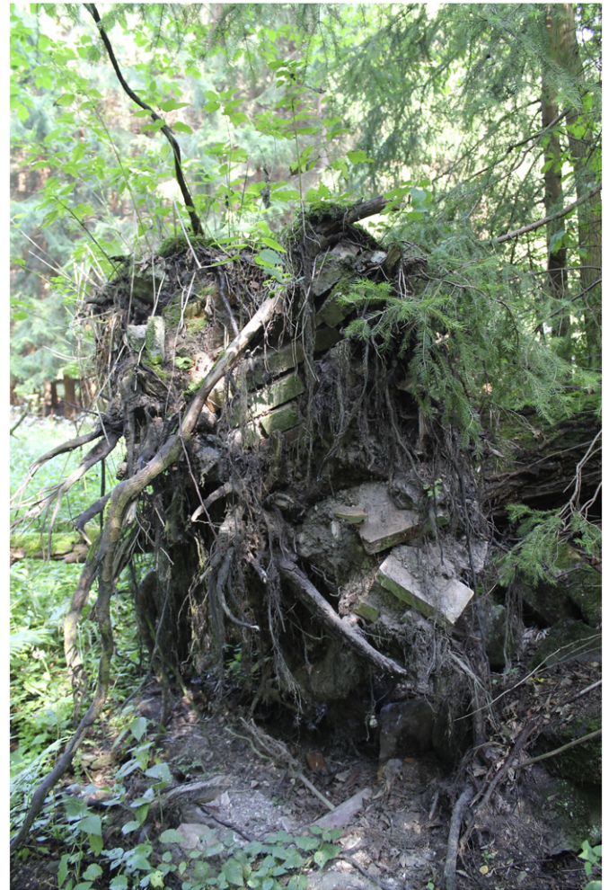
Fig. 12. Uprooted tree with bricks in a root plate. The tree was growing on the wall of an abandoned old house in the Table Mts., SW Poland. During uprooting event, it caused damage of the wall. (Photo: Ł. Pawlik).
